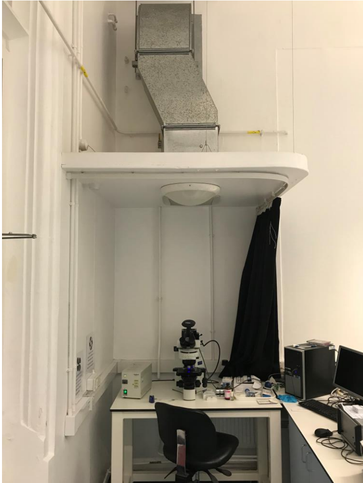
Figure 2. Extraction of mercury vapor must be accounted for when siting the microscope.
